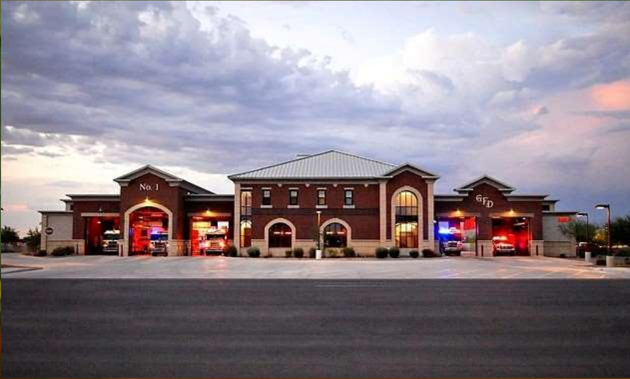
Gilbert Fire Station 1, Williams Field Road
